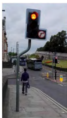
Traffic signal pole situated to the side of road reserve to allow for barrier free pedestrian access whilst light is still visible to vehicles. Applicable to all road signs and street lights.
