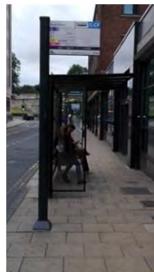
Bus shelter turned around to ensure safety of pedestrians requiring use of road reserve. Back of shelter is made from Perspex to still have visual access of traffic.
